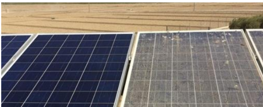
Example of extreme dirtiness compared to clean module
